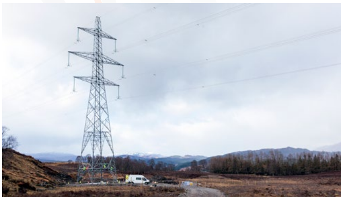
SHE Transmission has completed and energised its section of the Beaully – Denny 400kV replacement line between Beaully and the Wharry Burn
